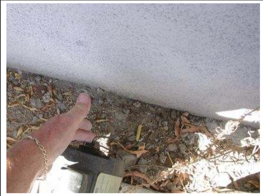
003. SC.E.2327. One pool pump motor has a ground wire that is loose at the ground lug.
